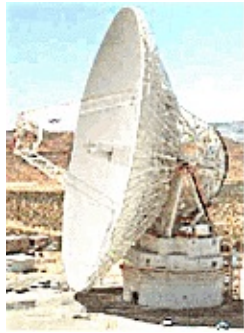
Figure 15.4: Deep Space Station 14 pointing its 70 m aperture toward the eastern horizon in the Mojave Desert.
