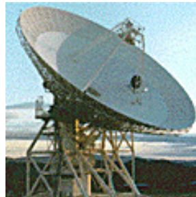
Figure 18.1: One of DSN's 34 m aperture Beam Waveguide Deep Space Stations.
