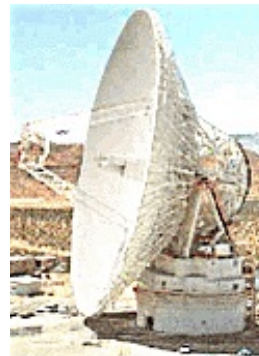
Figure 2.8: DSN station with AZ-EL mount (DSS-14).
