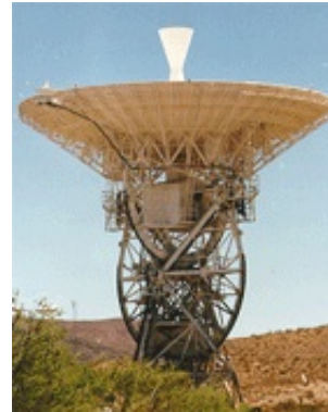
Figure 2.9: DSN station with X-Y mount (DSS-16).
