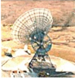
Figure 2.7: An older DSN station with HA-DEC mount (DSS-42).
