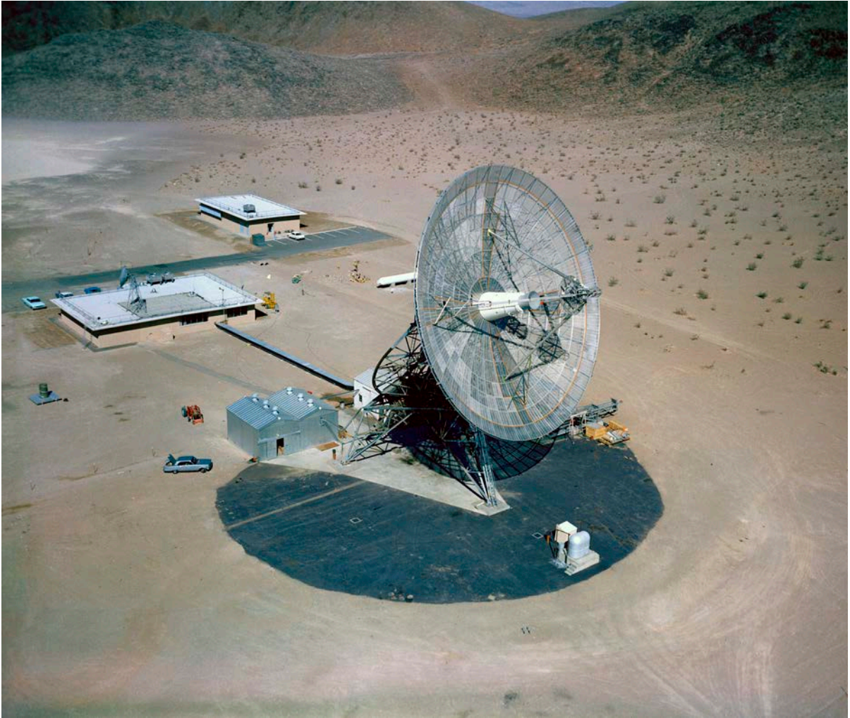
During the Pioneer IV mission, NASA tested a new space communications system. One component of the system was this 26-meter diameter antenna at Goldstone, California, the first of several antennas that would later constitute nodes in NASA's Deep Space Network. Credit: NASA/JPL-Caltech
