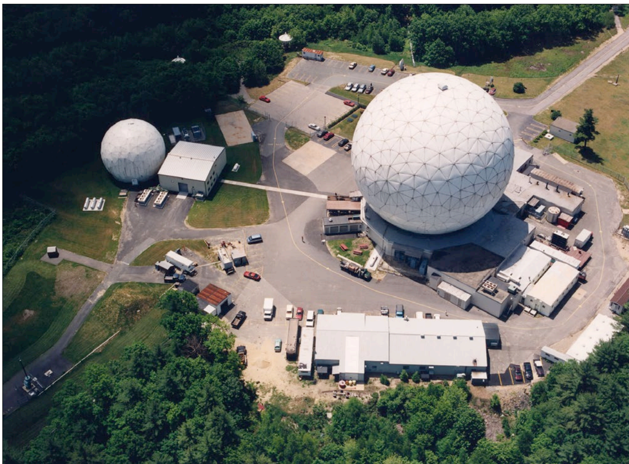
Figure 4. Millstone/Haystack radar complex used to track orbital debris. The installation is located in Tyngsboro, Massachusetts.
