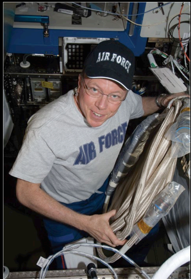
Figure 2. Astronaut Mike Fossum installs an electrical bypass jumper to provide a redundant power feed for the MBSU-1 in case the ISS had to be left uncrewed.
