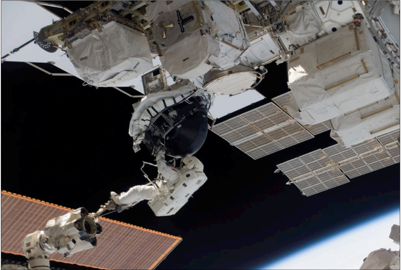
Astronaut Dave Williams carrying one of the four massive gyroscopes used to control the orientation of the International Space Station (ISS) during replacement operations on STS-118/ISS-13A.1 in August 2007. Williams (anchored in a foot restraint) is being moved along with the Control Moment Gyroscope (CMG) by the space station robotic arm. The CMG is being installed on External Stowage Platform-2 near the ISS airlock, where it was stored awaiting a return to Earth for refurbishment.
